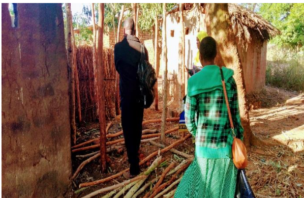
Goat shelter, under construction
